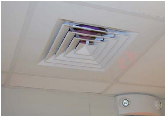
HVAC Vents Discharge
