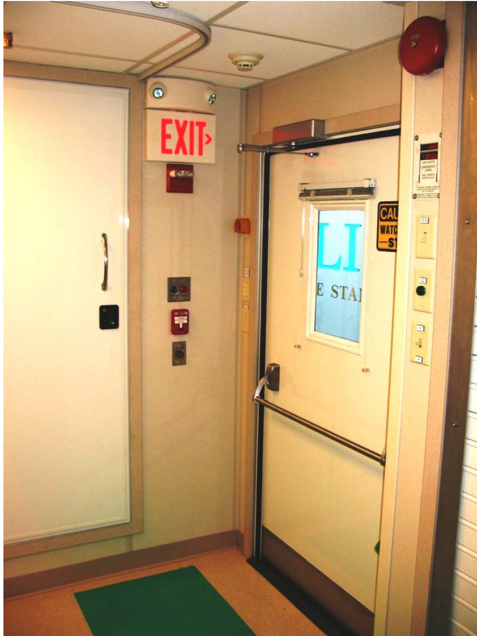
Figure 8: Exterior Staff Door
