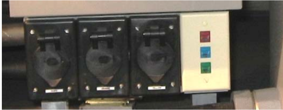
Figure 15: Phone & Data Line Connections
