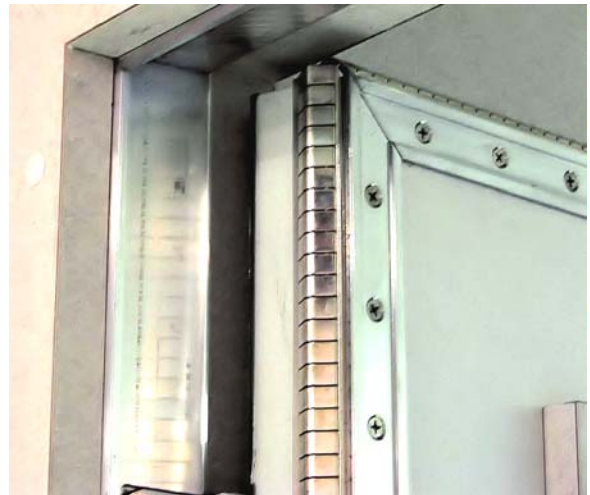
Close up of RF door trim Figure 61: RF Shielding
