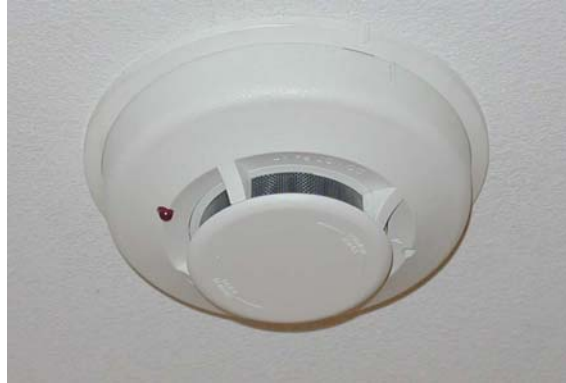
Figure 25: Smoke Detector
