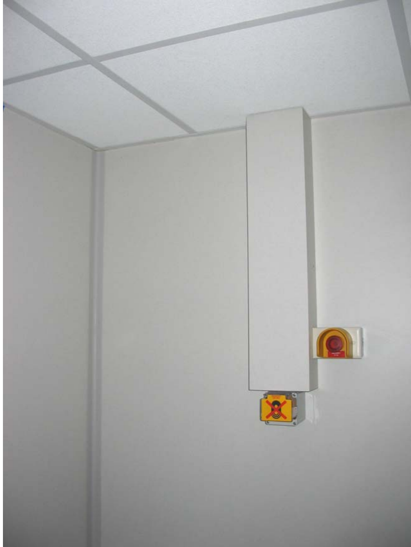
Left side wall behind magnet
