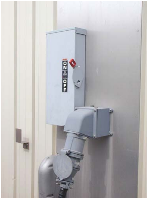
Figure 22: Shore Power Connection
