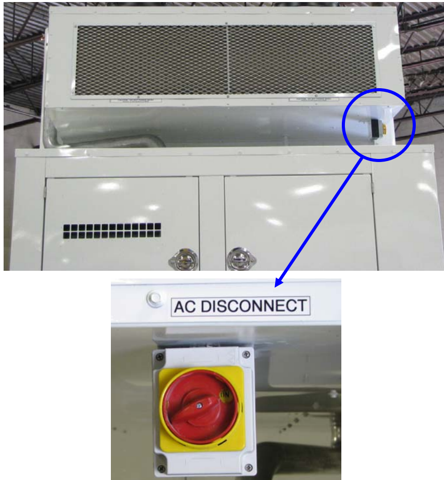
Figure 35: Northern Air A/C Units
