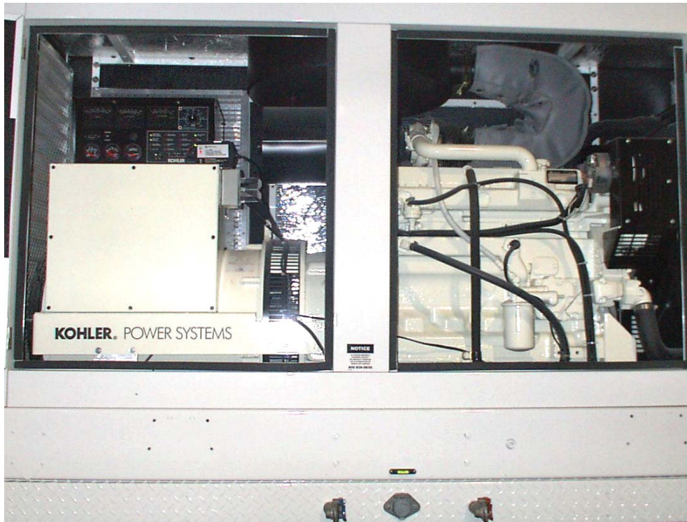
Figure 32: Generator Compartment
