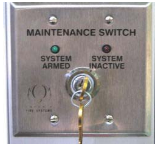
Figure 24: Maintenance Switch
