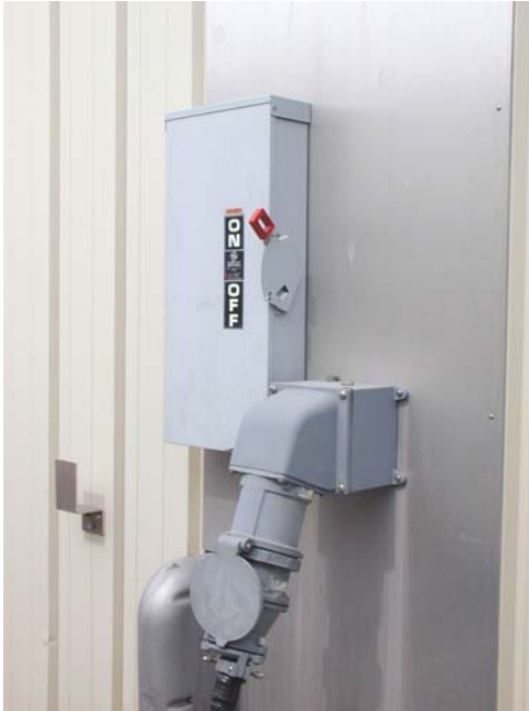
Figure 31: Shore Power Connection
