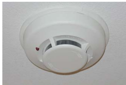
Figure 18: Smoke Detector
