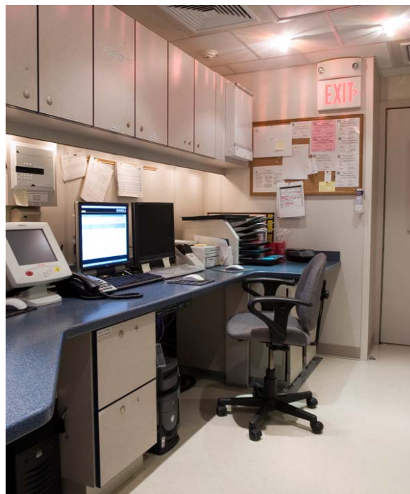
Figure 3: Control Room Overall
